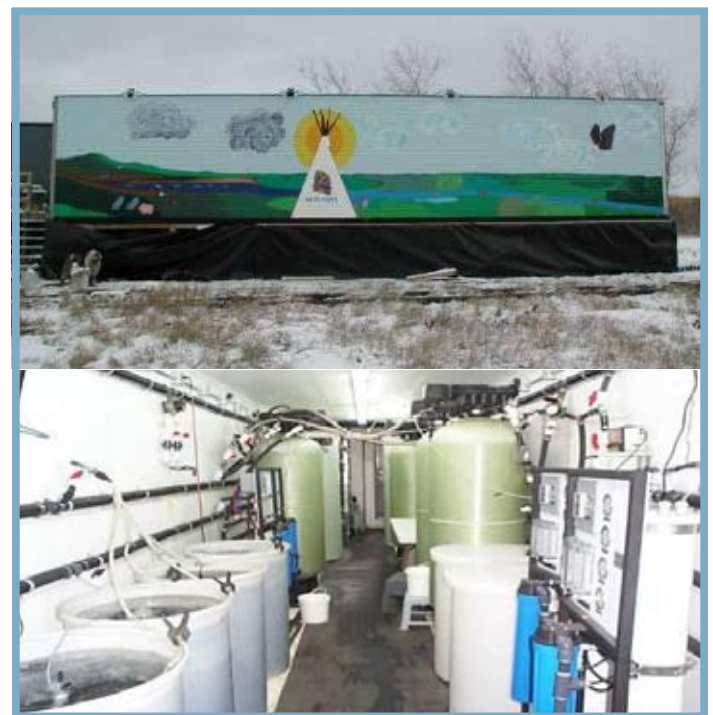
Fig. 4. The pilot water quality trailer (outside top and inside bottom) used by Yellow Quill First Nation to test raw water treatment processes.
