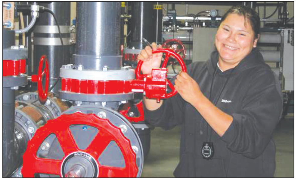
Roberta Neapetung setting a valve in the new IBROM plant.
